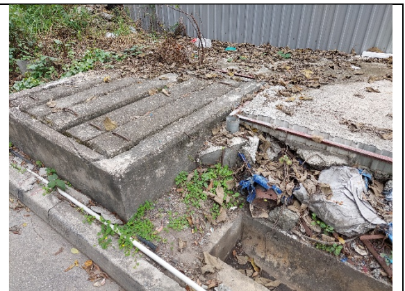
Plate No. 4 – Existing Catchpit 1 and the adjacent existing U channel which is separated from the Existing Catchpit 1 and conveys flow toward Castle Peak Road – Hung Shui Kiu
