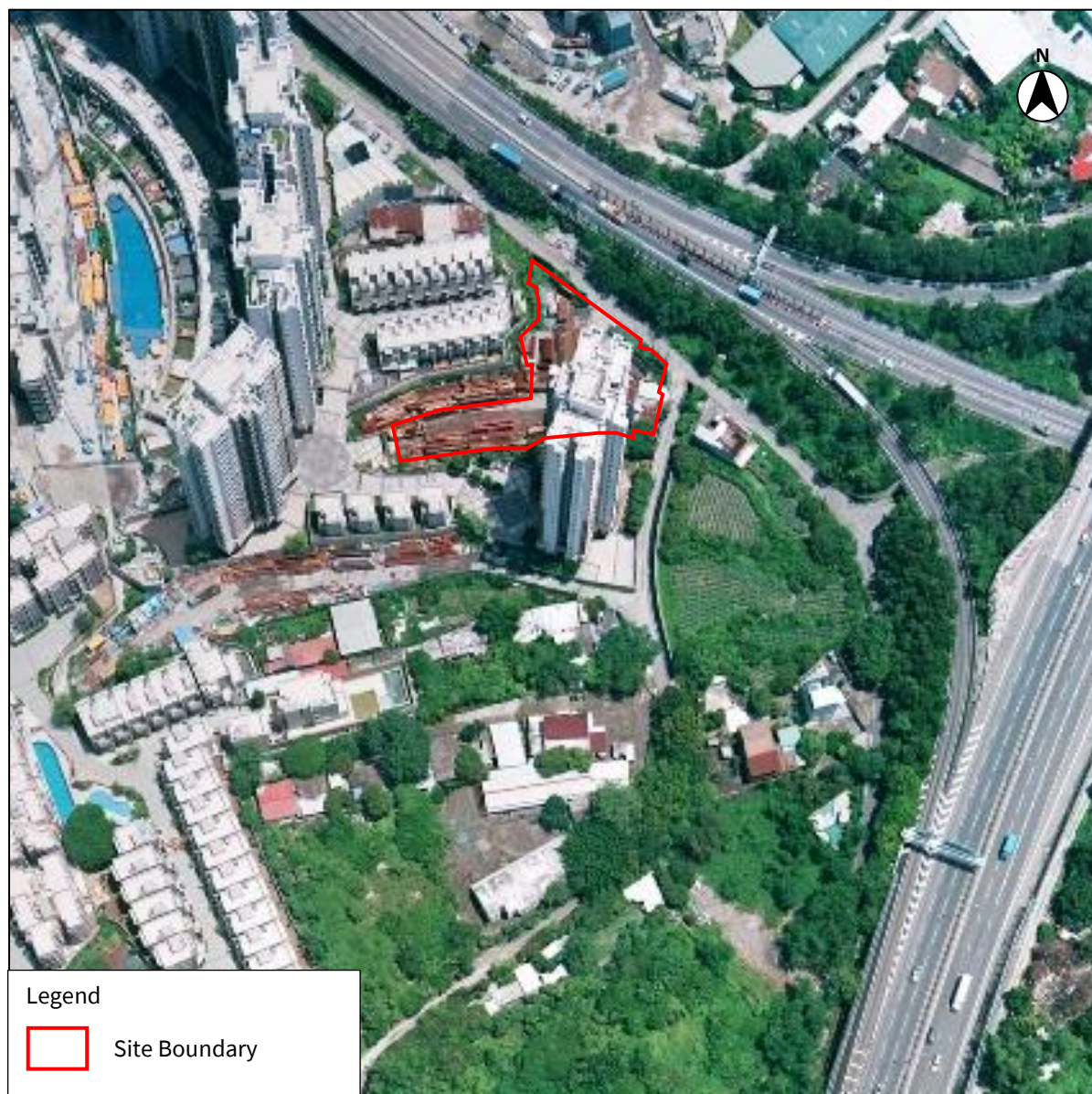
Figure I-6 Aerial Photograph in Year 2014 (Photo No.: CW107934)
