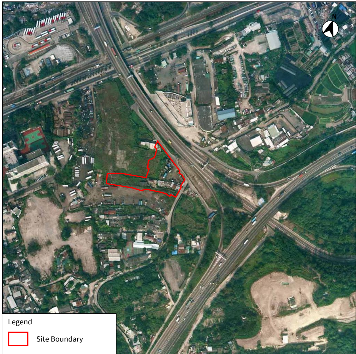
Figure I-5 Aerial Photograph in Year 2003 (Photo No.: CW54027)
