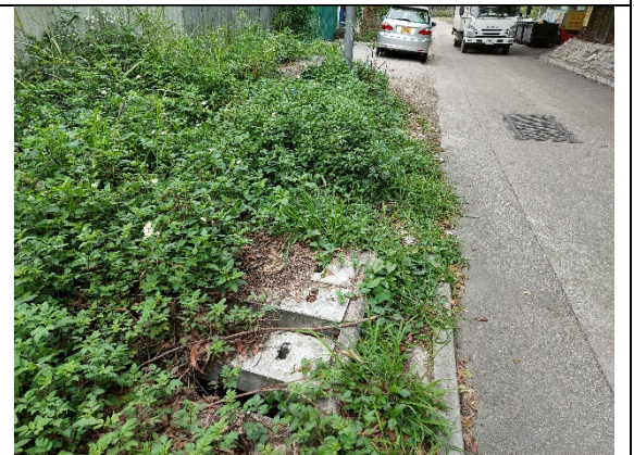
Plate No. 6 – Existing Catchpit 2 which should receive flow from an existing 450U channel and discharge into an existing 525mm diameter drain with respect to the GEOINFO Map
